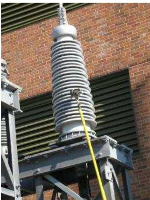
Figure 21 – Use of the hook stick in defect localization.
